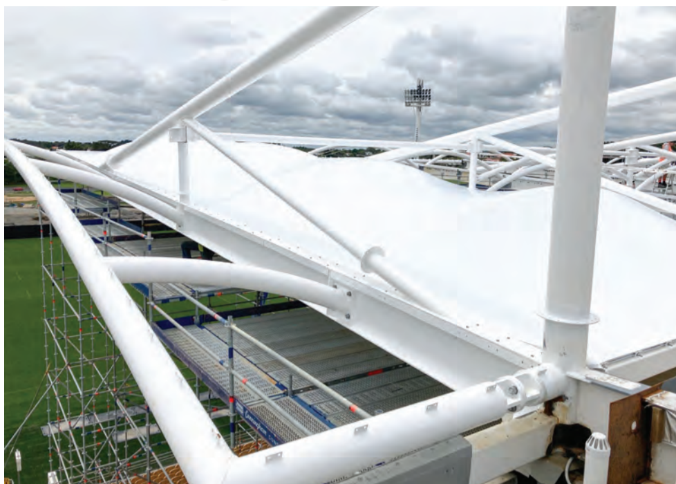
Yarrow Stadium roof November 2022.
